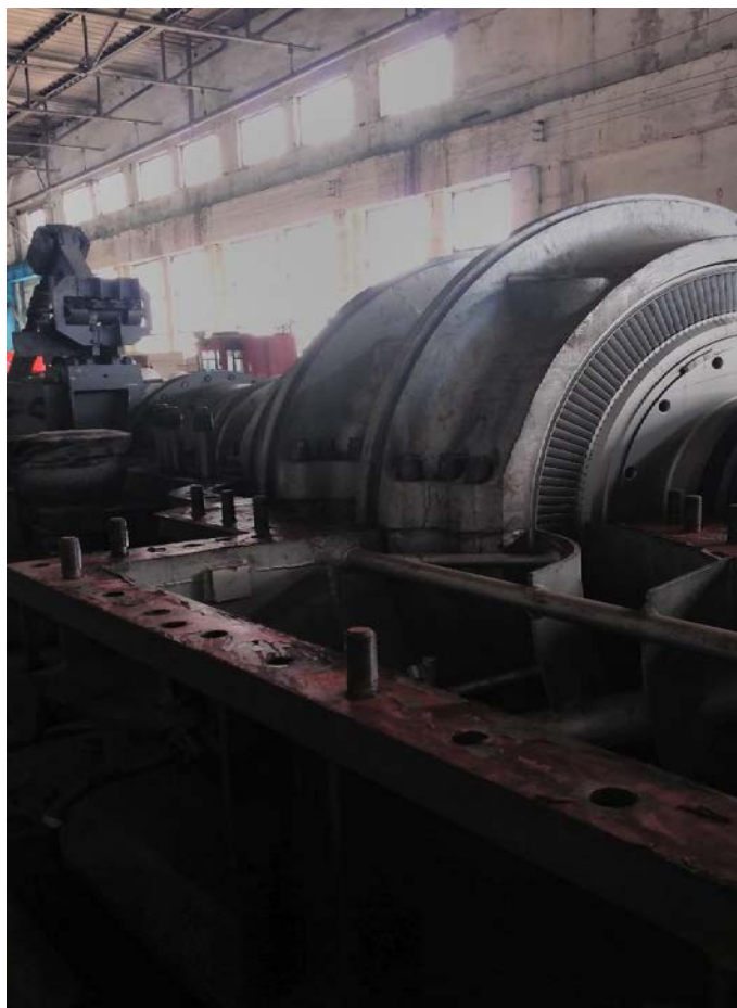
Photo 3 of the turbo-generator number 2 at CHP-3.
