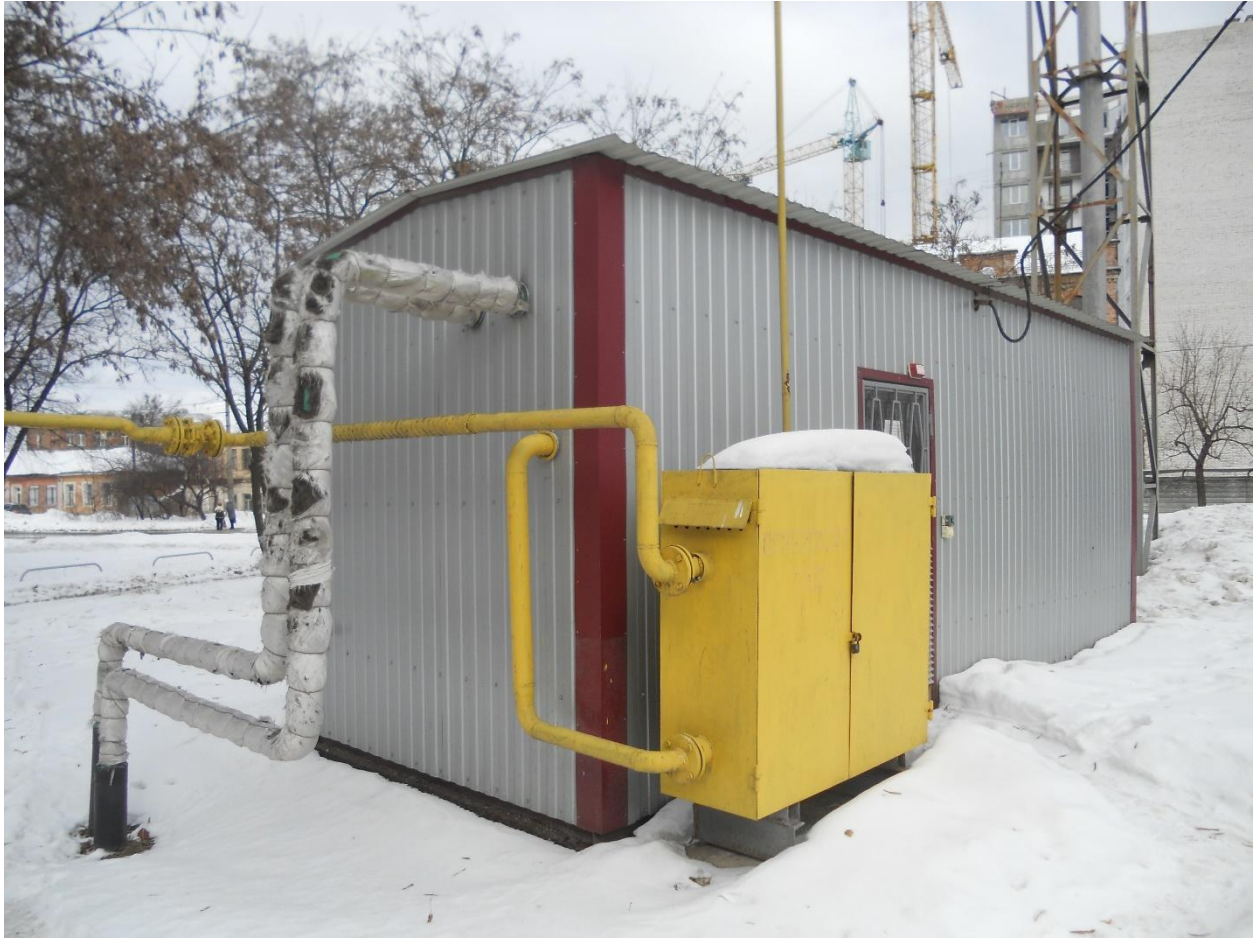
Photo 1 of a block-modular boiler-house (BMB)
